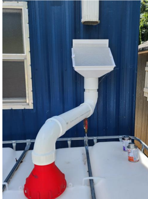
Figure 10. PVC inlet connecting leaf particulate filter and 3D printed lid adapter attached to home using preinstalled gutter fastenings.
