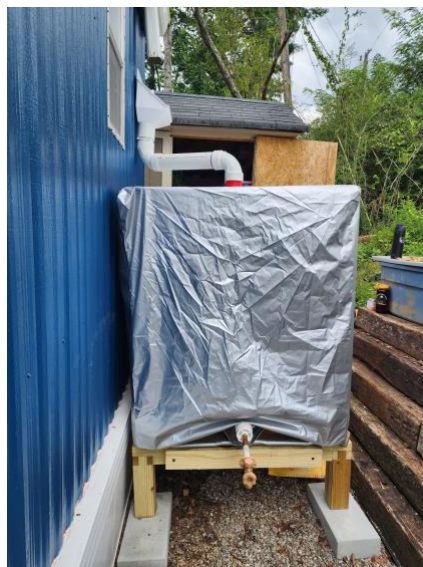
Figure 12. First prototype installed under a home gutter system using the cradle system.
