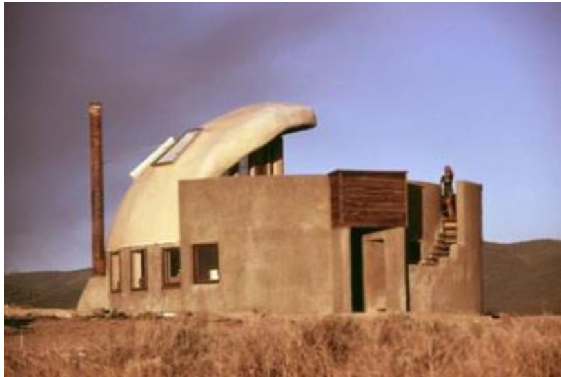
Figure 6. Mike Reynolds, architect, 1975, Earthships Biotecture , EXPERIMENTAL HOUSE COMPLETED NEAR TAOS, NEW MEXICO USING EMPTY STEEL BEER AND SOFT DRINK CANS - NARA - 556623" by David Hiser, 1937-, Photographer (NARA record: 3651517) - U.S. National Archives and Records Administration.
