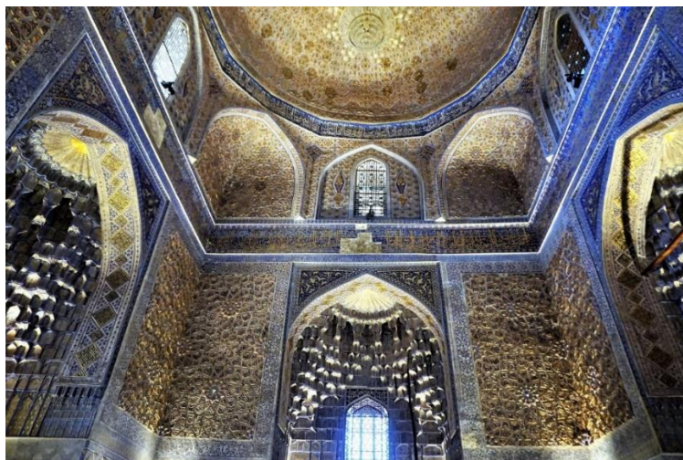
(Preceding Page) Figure 10. Part of lower wall, transition zone, and inner dome.
