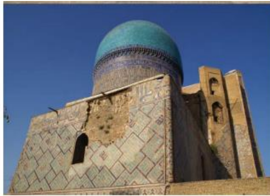
Figure 8. Missing Kufic script due to broken gutters https://www.silkroadfoundation.org
